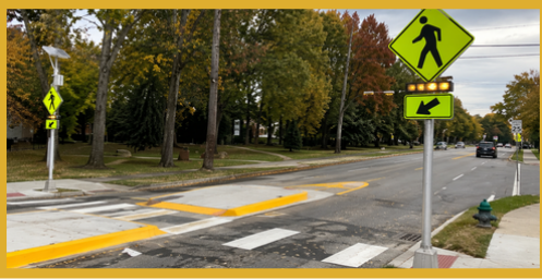
Rapid Flashing Rectangular Beacons (RRFB)
