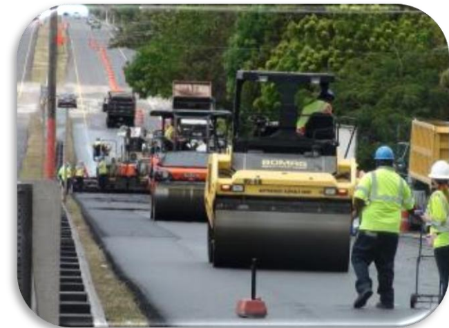
Laydown and compaction of WMA, Yauco, PR-Betterroads Asphalt Corp. (April 8, 2011)
