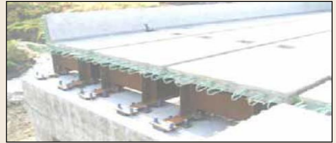
Alt. 2: Steel girder with integrated concrete deck
