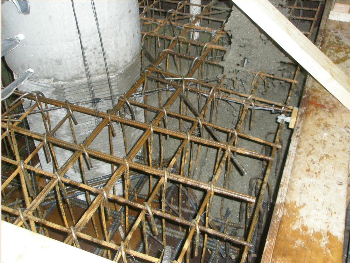
Footing Connection: Construction
