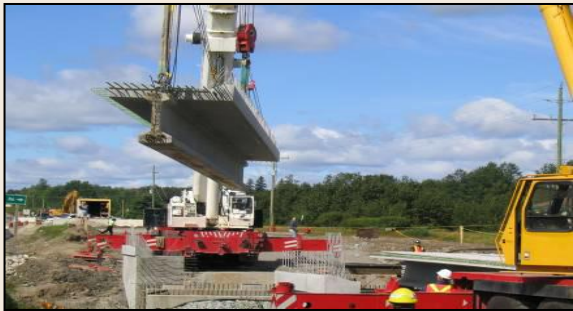
Alt. 3: AASHTO beams with integrated concrete deck
