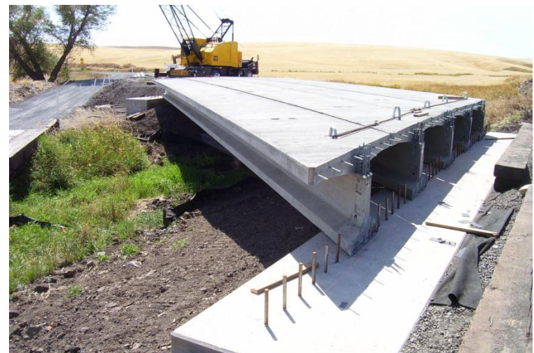
Fig. 7: Adjacent Deck Bulb Tees ( www.cprestress.com )
