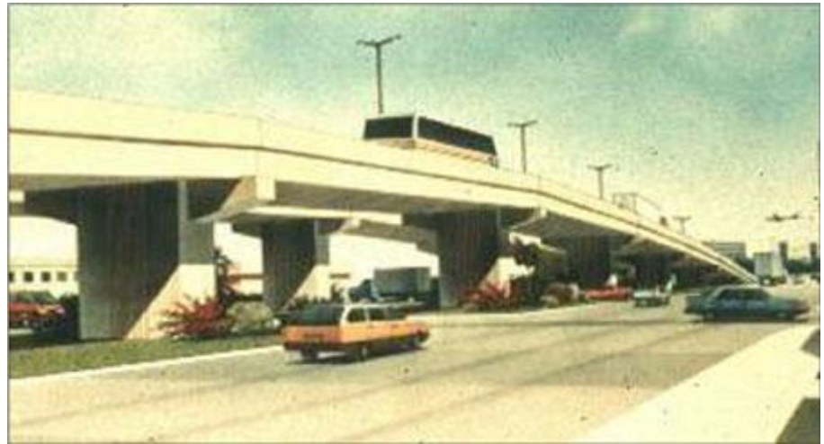
Fig. 29: Baldorioty de Castro Avenue Bridge in San Juan, PR ( www.fhwa.dot.gov )
