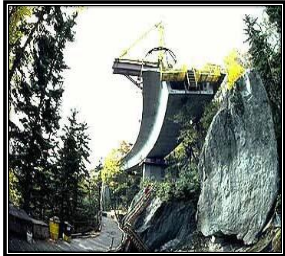
Fig. 18: Linn Cove Viaduct, NC ( www.fhwa.dot.gov )
