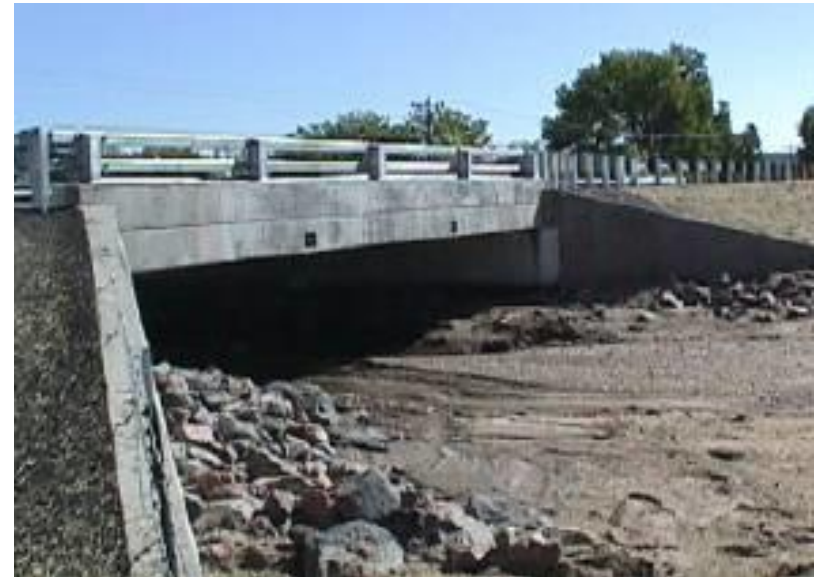
Fig. 27: Colorado Department of Transportation's Highway 86 Bridge over Mitchell Gulch ( www.fhwa.dot.gov )
