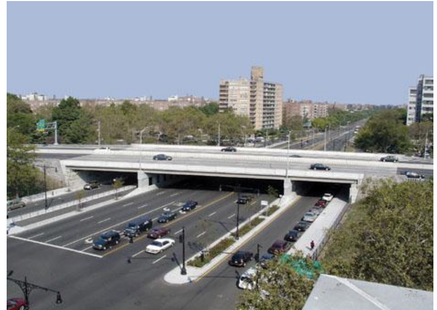
Fig. 28: New York City Department of Transportation's Belt Parkway Bridge over Ocean Parkway ( www.super-slab.com )
