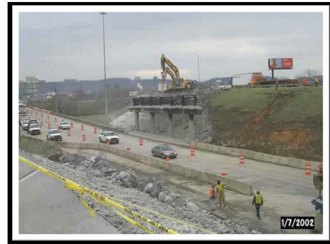
Fig. 16: I-59 and I-65 Interchange, AL ( www.fhwa.dot.gov )
