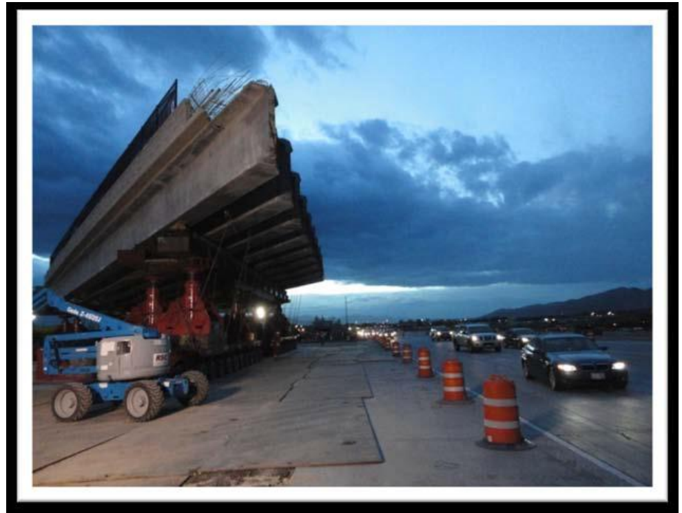
Fig. 11: Superstructure Span on SPMT ( www.fhwa.dot.gov )
