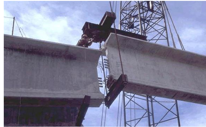
Fig. 6: Precast Spliced Tub Girder( www.adaptsoft.com )
