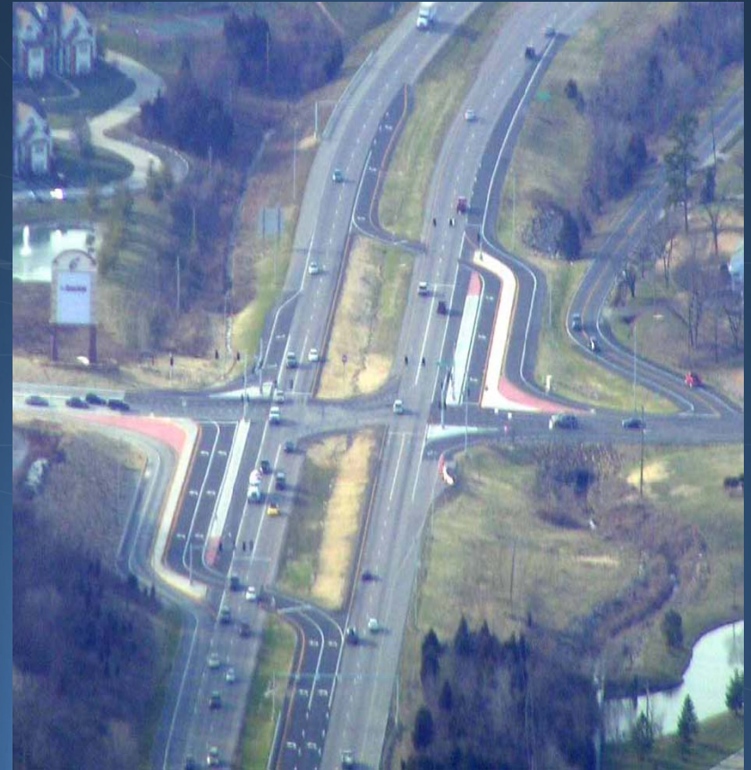
DLT intersection at the intersection of U.S. Route 30 and Summit Drive in Fenton, MO.
