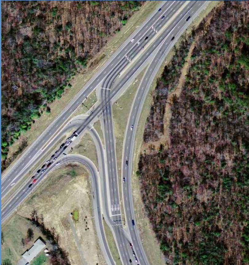
DLT intersection at the intersection of Indian Head Highway (MD 210) and Berry Road (MD 228) in Accokeek, MD.
