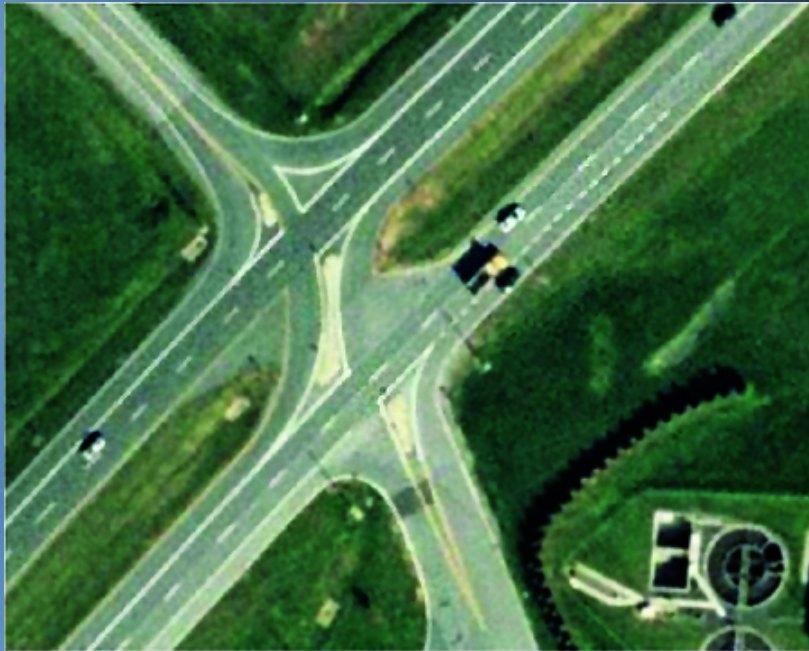
U.S. Route 15 RCUT intersection in Emmitsburg, MD. Source: FHWA
