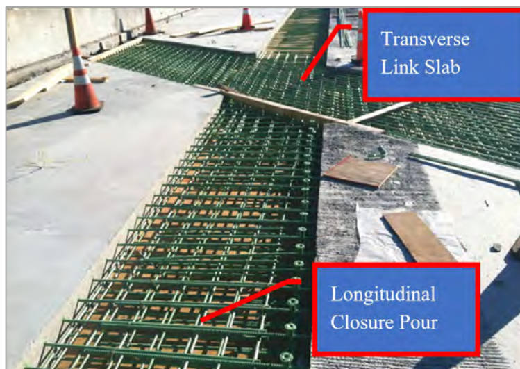
Figure 11. Photo. Construction of Transverse Link Slab and Longitudinal Closure Pour Between Precast Deck Segments.
