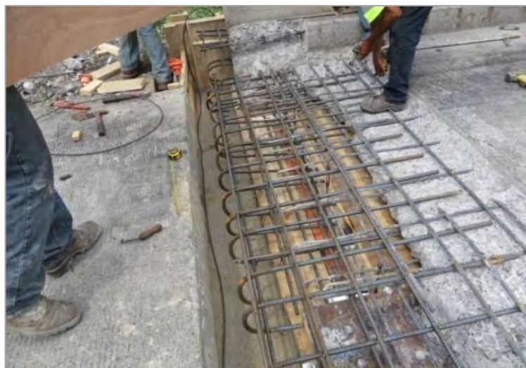
Figure 10. Photo. VDOT Deck Slab Extension Installation at Abutment.
