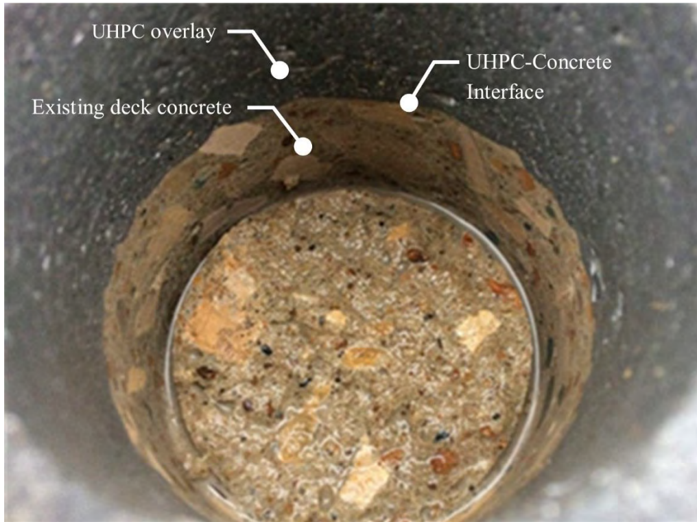
Figure 32. Photo. Core location for specimen G2-9.
