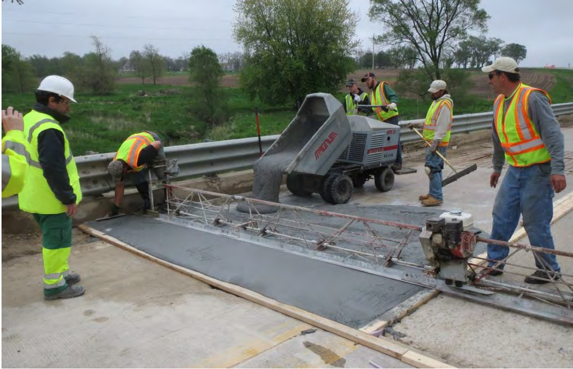
Figure 19. Photo. Placement of the UHPC overlay on the westbound lane.
