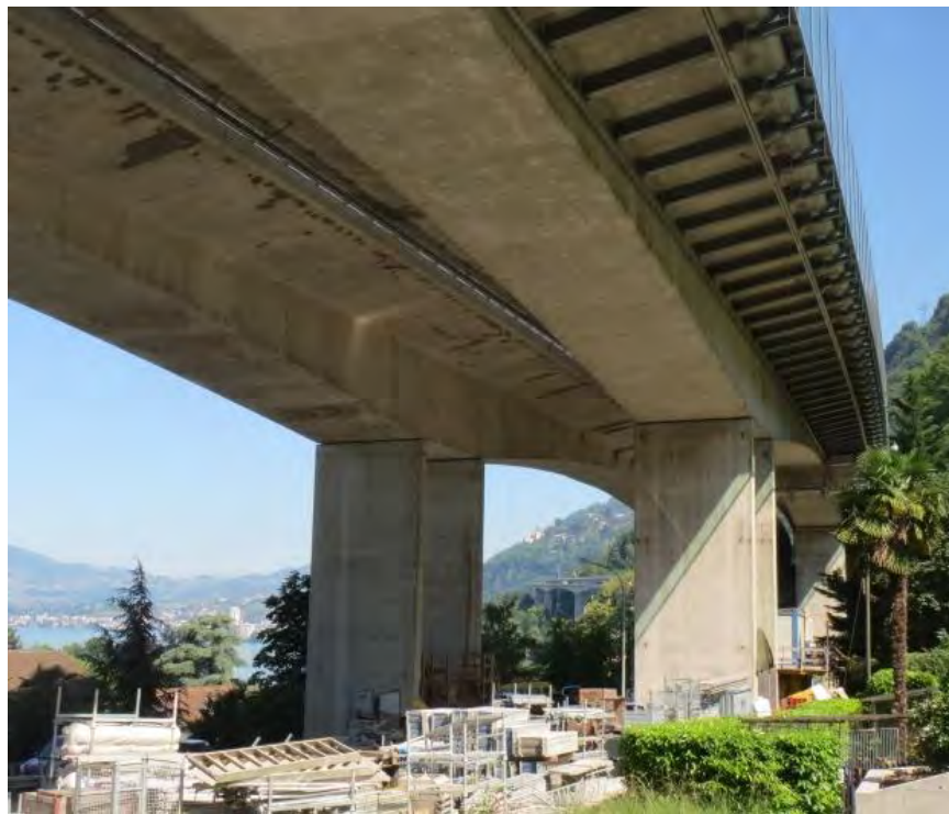
Figure 10. Photo. Chillon Viaduct: Parallel post-tensioned box girder structures.
