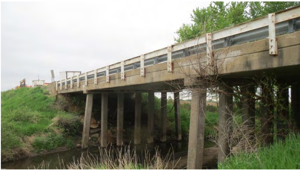
Figure 14. Photo. Laporte Road bridge.
