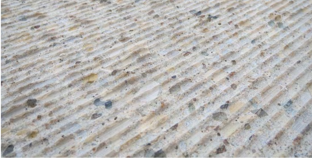
Figure 18. Photo. Deck surface after scarification.
