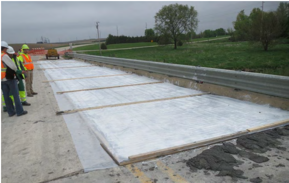
Figure 20. Photo. Curing of the overlay on the westbound lane.
