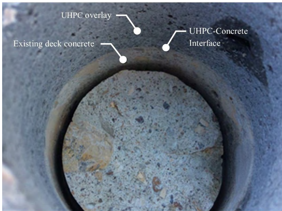
Figure 38. Photo. Core location for specimen G3-13.
