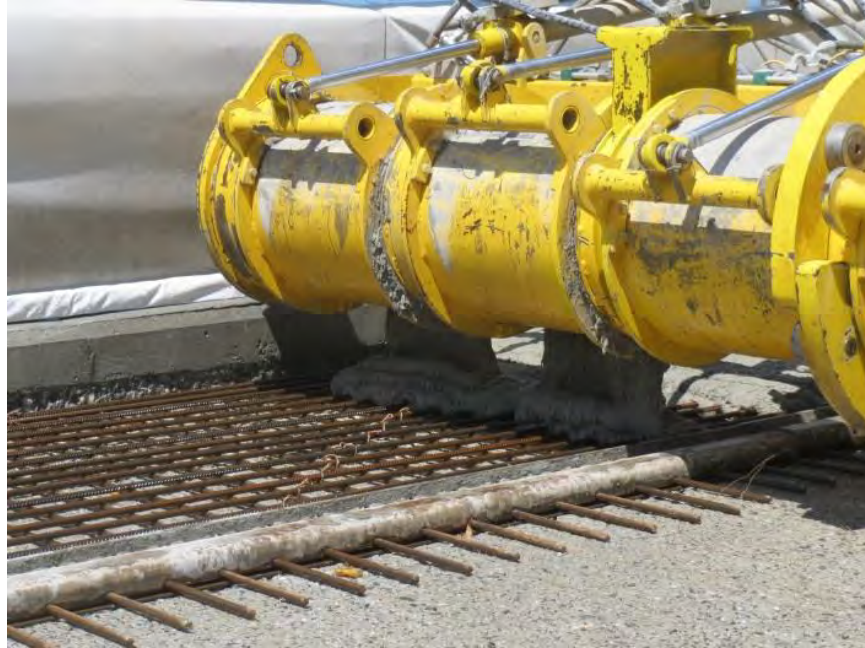
Figure 13. Photo. Placement of UHPC in the Chillon Viaduct project.
