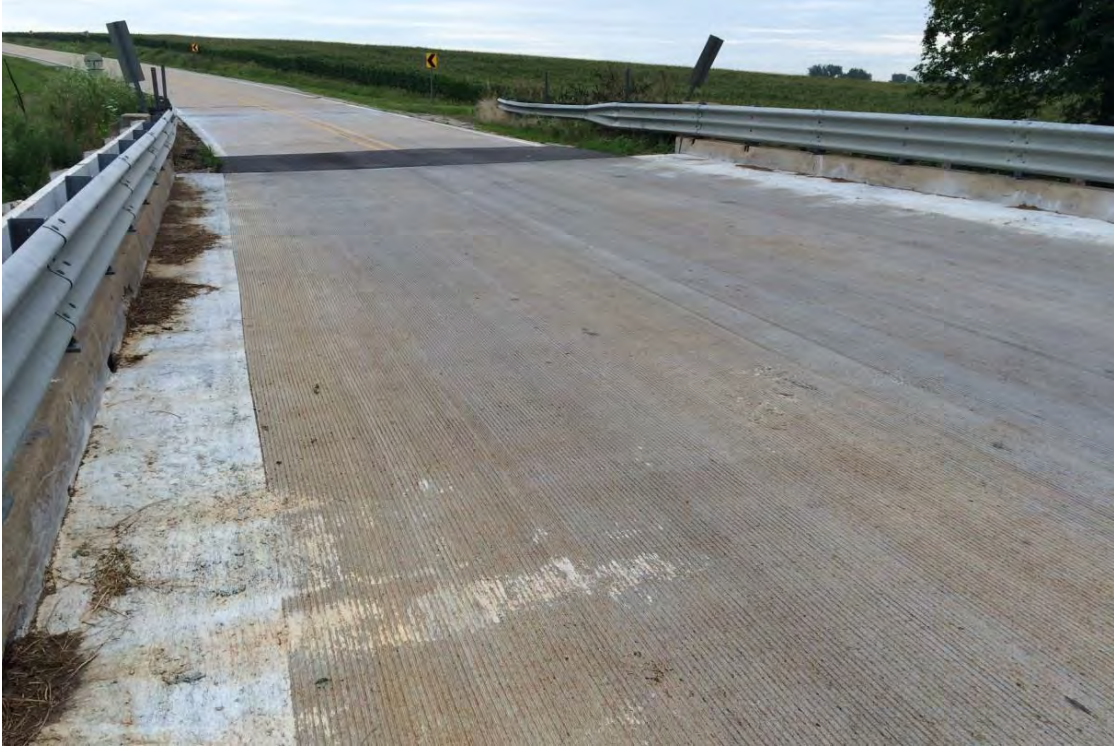
Figure 21. Photo. Completed overlay after deck milling looking eastbound.
