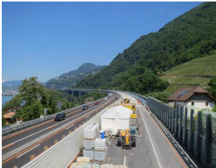
Figure 12. Photo. Aerial view of the Chillon Viaduct UHPC overlay construction project.
