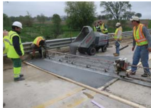
Figure 10. UHPC overlay installation on the westbound lane. (2)
