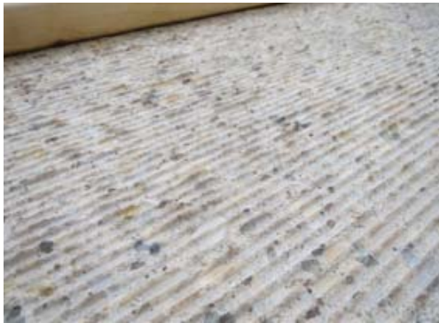
Figure 9. Deck surface after diamond grinding. (2)
