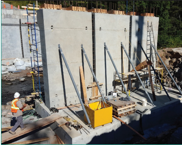
Figure 8. Photo. Precast abutment wall segments to be connected with UHPC on Rang Saint-Georges Bridge in Quebec, Canada.
