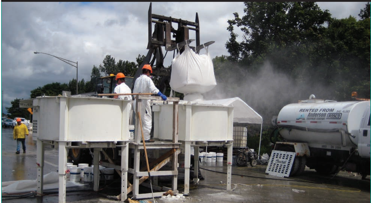
Figure 27. Photo. Mixing operation for the field-cast UHPC. (25)
