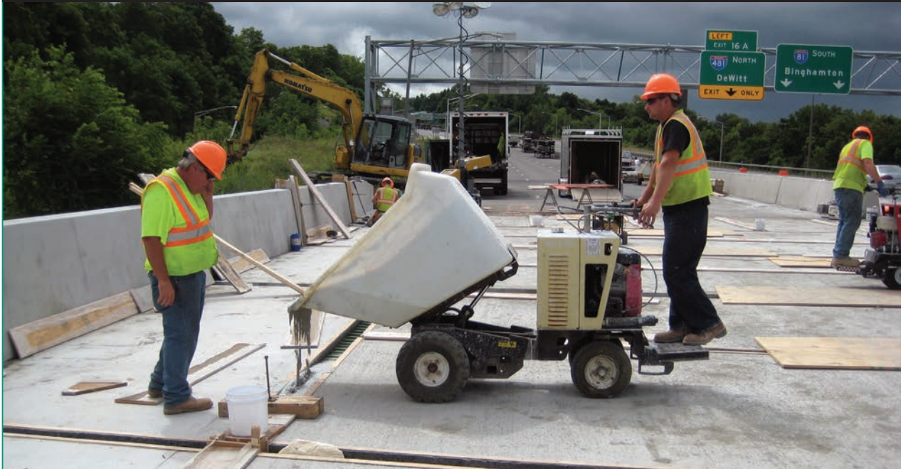
Figure 28. Photo. Placing operation for the field-cast UHPC. (25)
