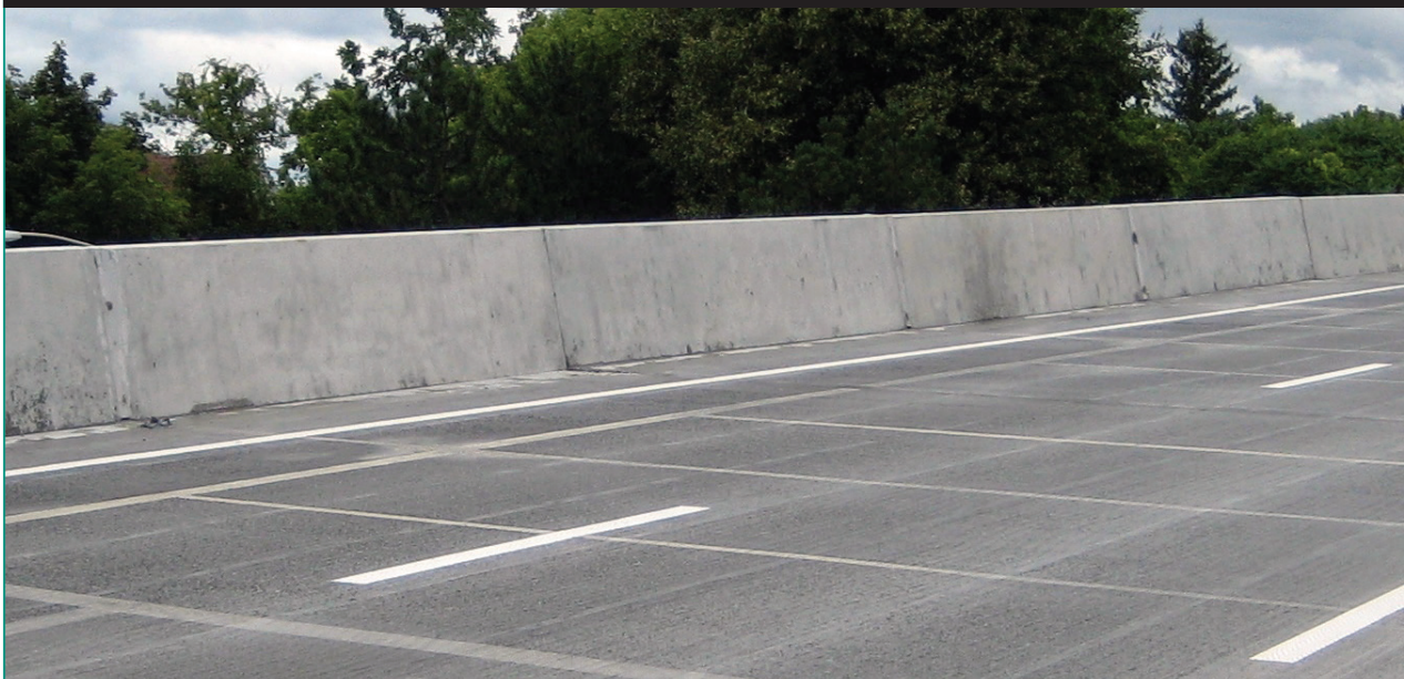
Figure 29. Photo. Bridge deck after grinding, grooving, and opening to traffic. (25)
