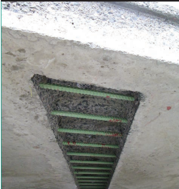
Figure 24. Photo. Connection detail on underside of precast deck panel. (25)
