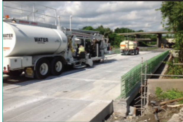
Figure 17. Photo. Surface profiling of a bridge deck on I-690 near Syracuse, NY.
