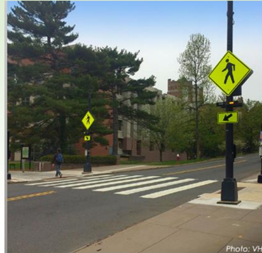
Crosswalk Visibility Enhancements
