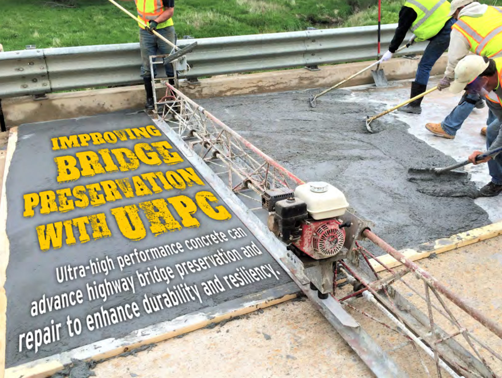
Ultra-high performance concrete (UHPC) has long been used for new construction in connections between prefabricated bridge elements. In the last few years, its use in bridge repair and preservation has increased as well. Here, crews install the first U.S. deployment of UHPC as a bridge deck overlay on a reinforced concrete slab bridge located in Brandon, IA, completed in May 2016.
