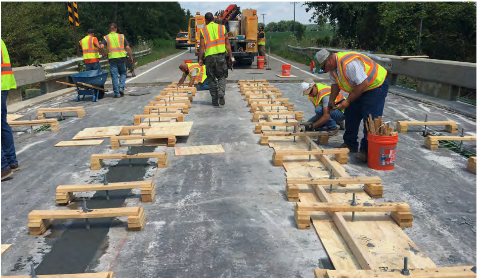
In 2017, the St. Clair County Road Commission in Michigan was the first to deploy an open-source UHPC mixture on a U.S. bridge. UHPC was used to repair the joints between the bridge's precast double T-beams.
