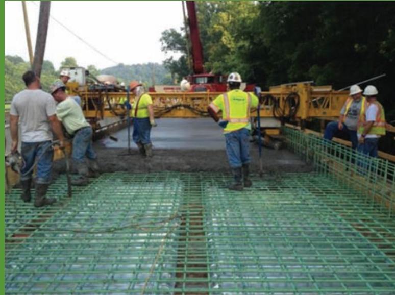
Figure 2. Internally cured bridge deck being placed in 2013 on US 150 over Lost River in Orange County, Indiana. Source: Barrett, T. J., Miller, A. E., & Weiss, W. J. (2015).
