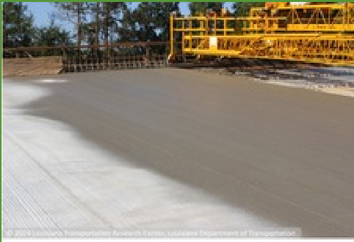
Figure 3. Internally cured bridge deck placed in Louisiana. Source: LTRC & LDOT
