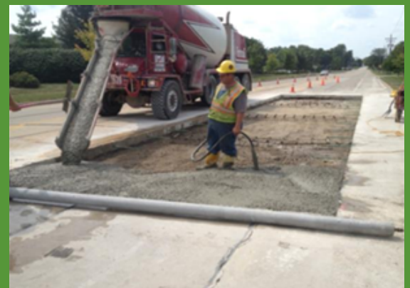
Figure 1. Internally cured concrete being used for concrete pavement patching Source: CP Tech Center
