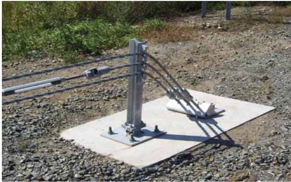
Three-Strand Cable Terminal
