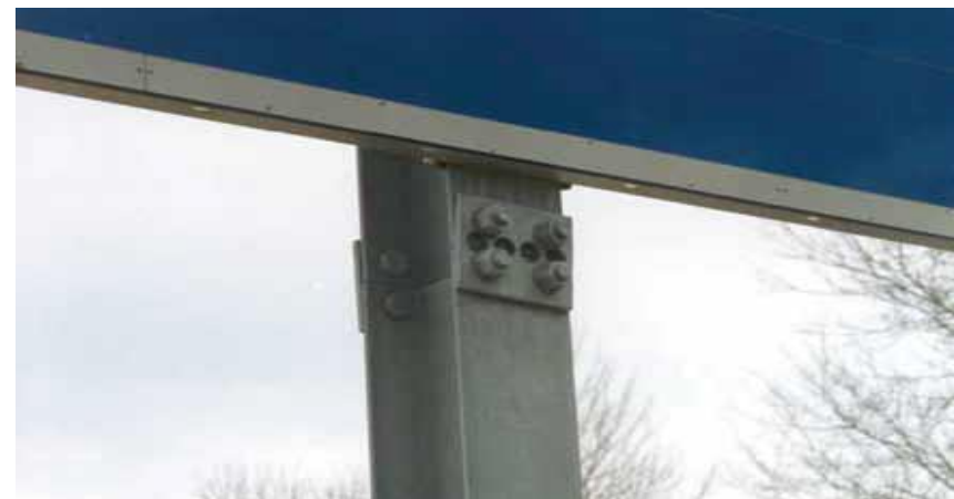
Perforated Fuse Plate Design
