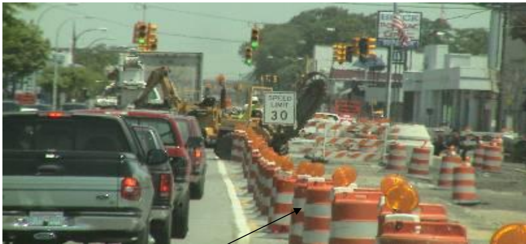
Flexible barrier separating traffic lanes and work area
