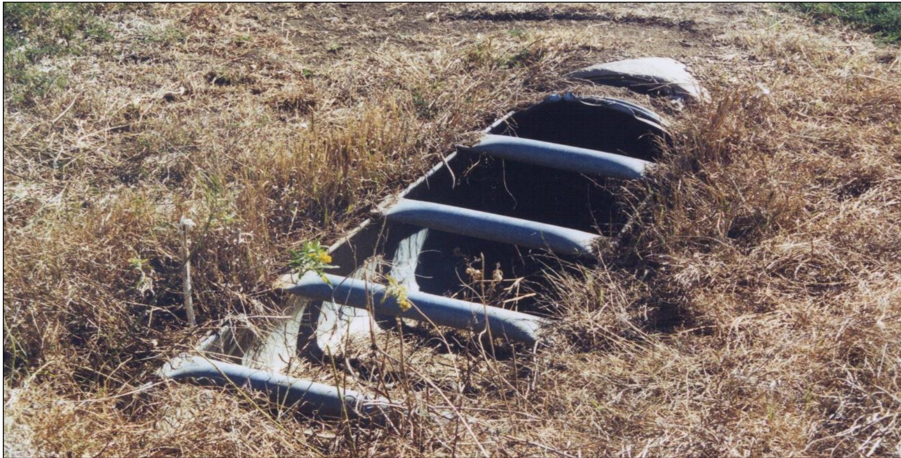
Safety Treatment for Parallel Drainage Pipe
