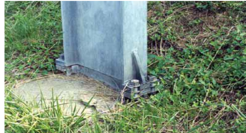
Typical Unidirectional Slip Base
