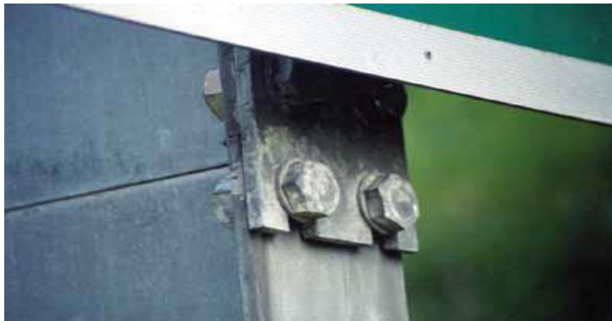
Slotted Fuse Plate Design
