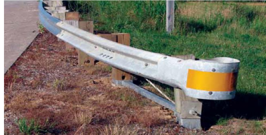
Flared W-Beam Terminals: Eccentric Loader Terminal (ELT)
