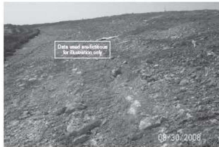
Rough slope trimming at SW side
