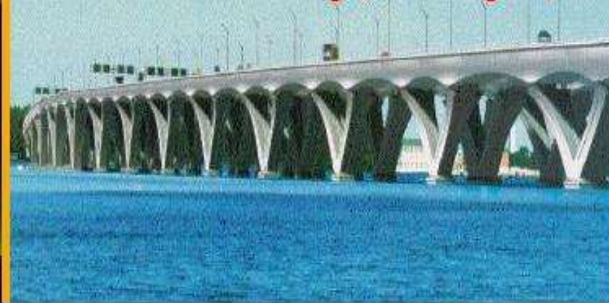
Woodrow Wilson Bridge, Washington, DC
