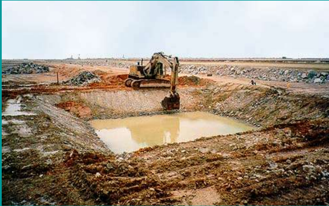
A Very Large Trial Pit
