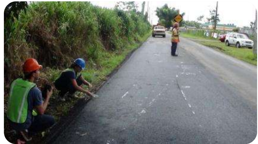
Verifying the 30° safety edge angle at paving project, Yabucoa, PR
