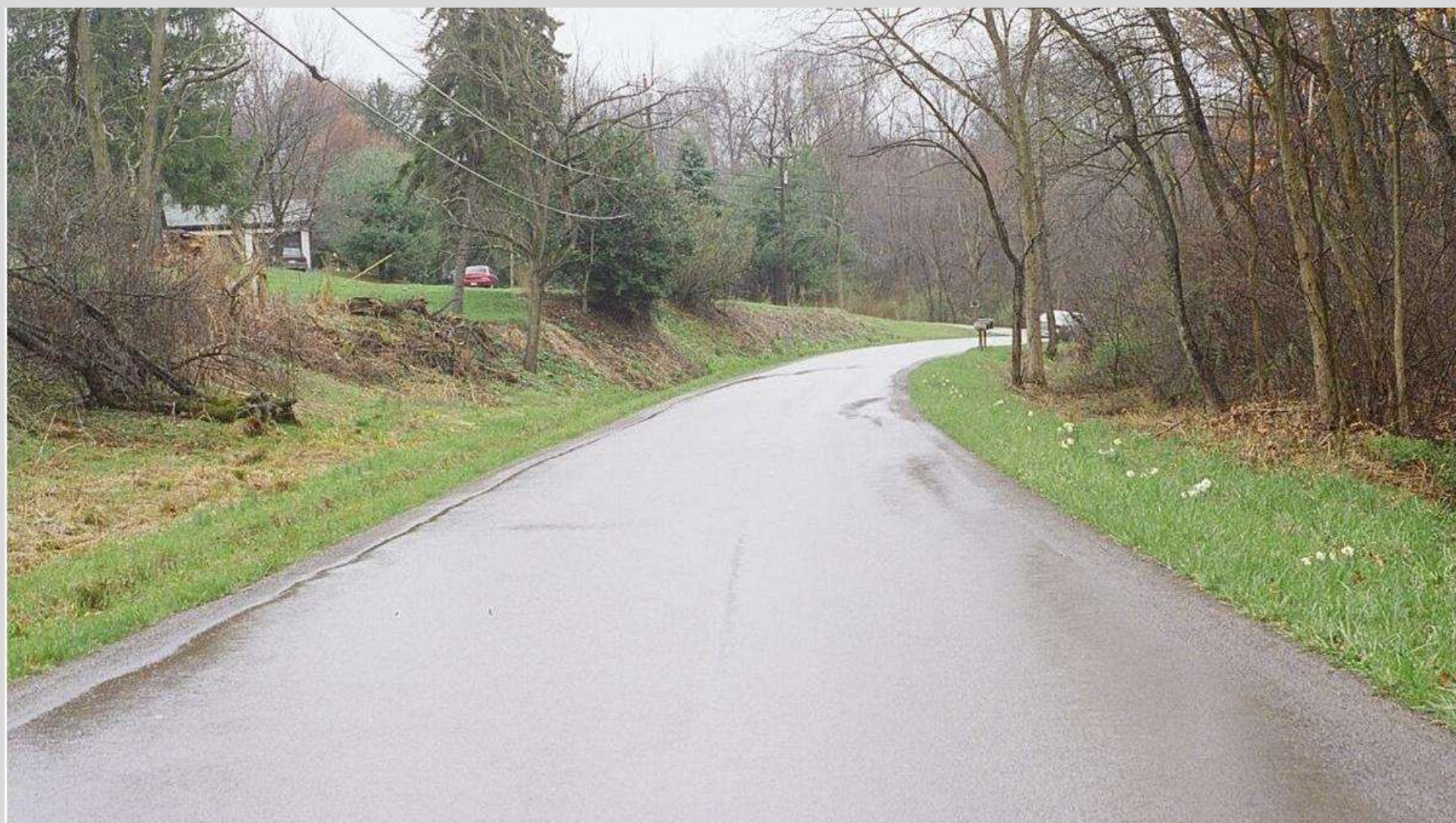
Example 1-Southbound View from Upstream of Curve
