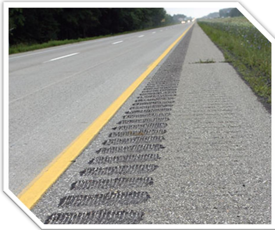
Rumble Strips and Rumble stripes
