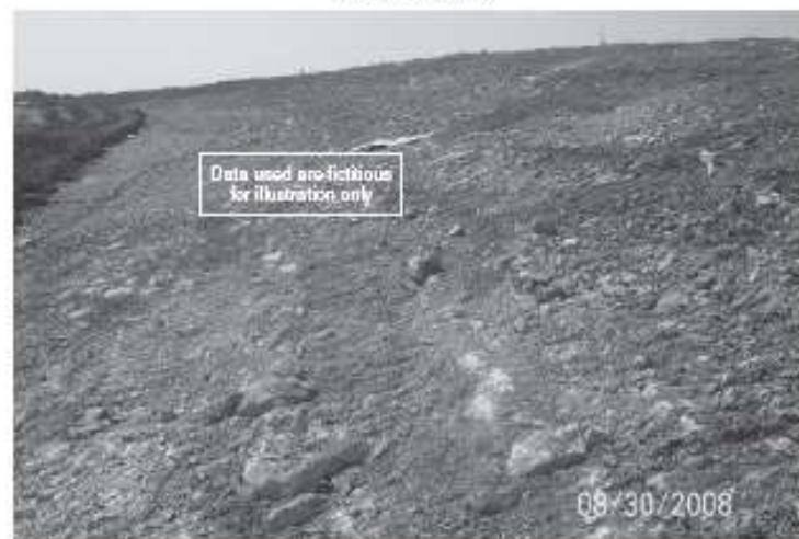
Rough slope trimming at SW side
