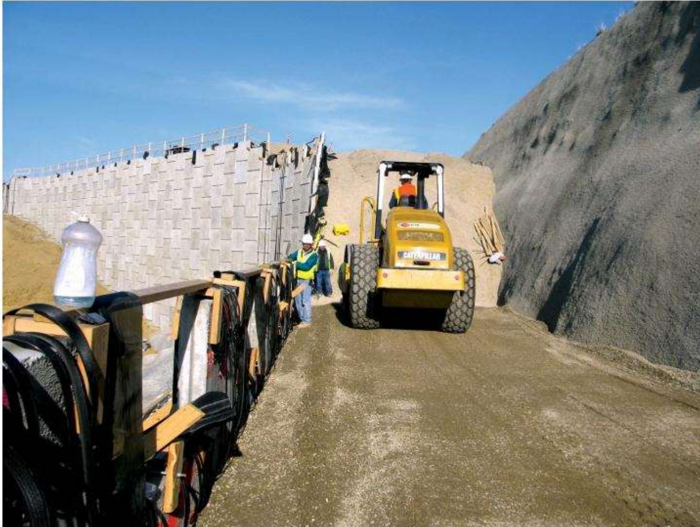
Figure 8 Construction of MSE wall 2. Photos courtesy of the authors
