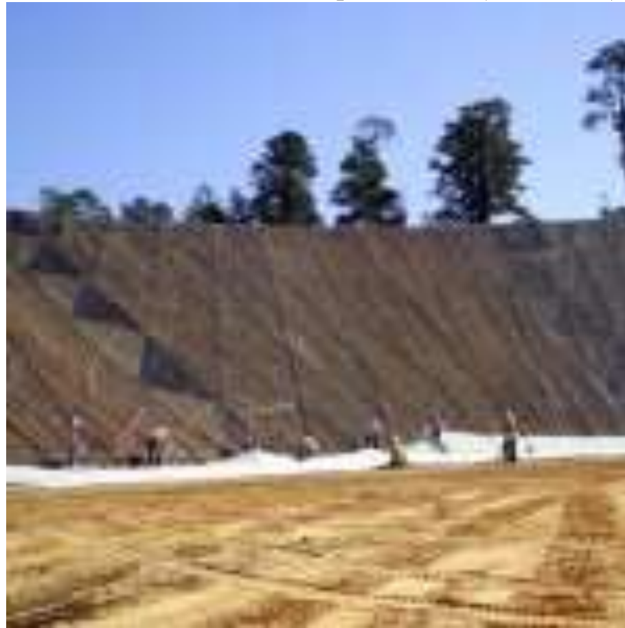
Reinforced Soil Slope using Geogrids
