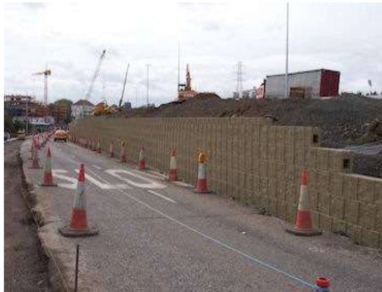
Modular Block Retaining Wall
