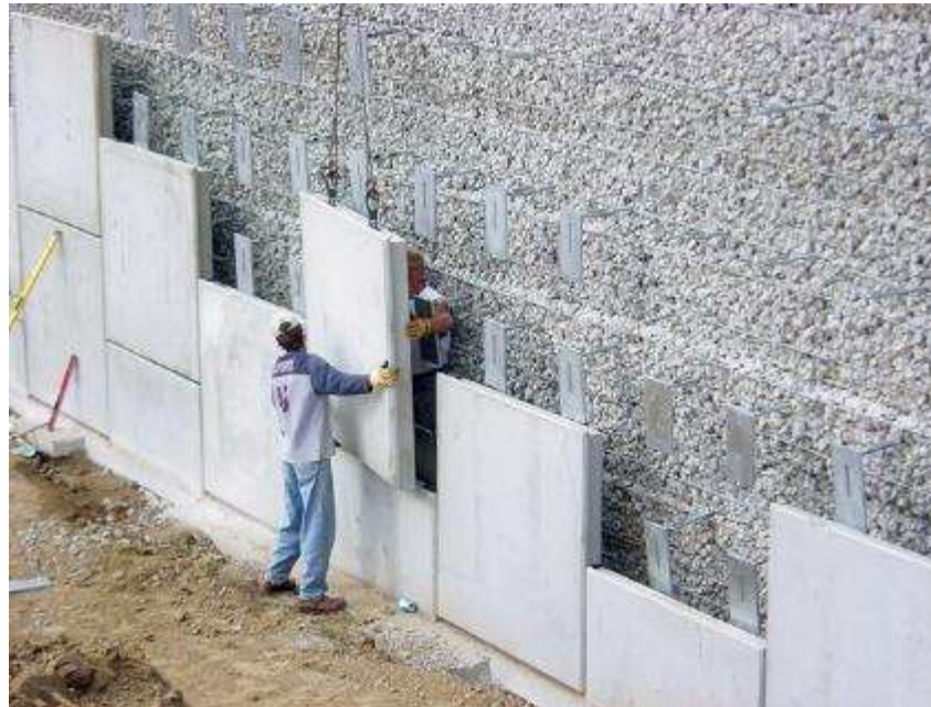
Precast concrete panels
