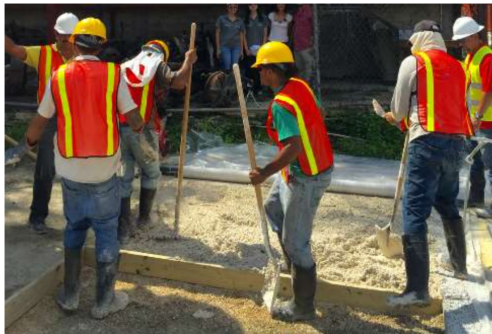
HDPE curing sheet (Star Ready Mix)
