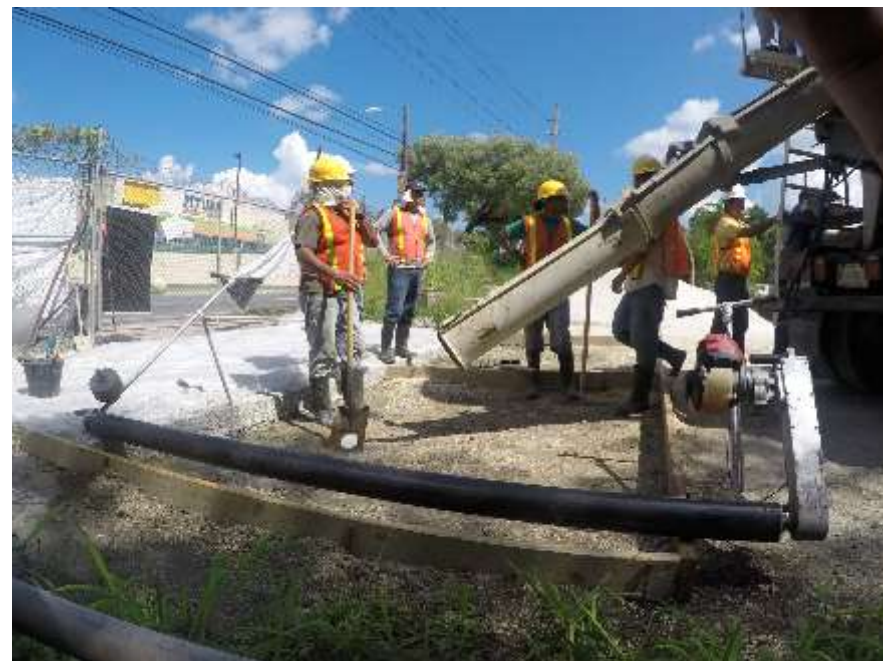
Shown here is a motorized roller screed (Star Ready Mix)
