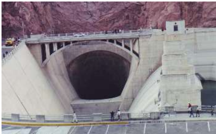
Hoover Dam spillway tunnel repair 1942
