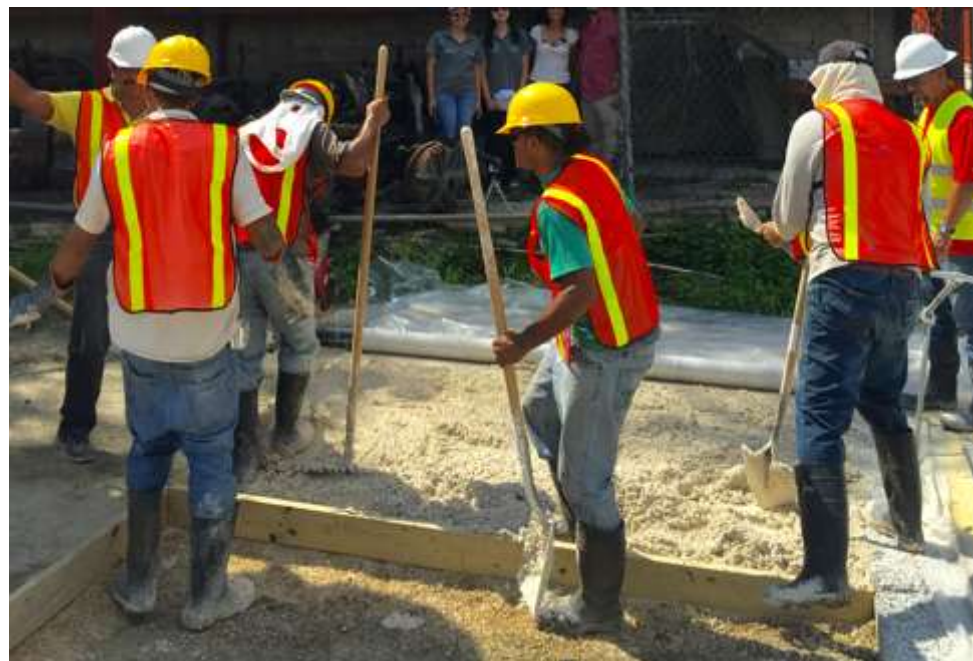
HDPE curing sheet (Star Ready Mix)
