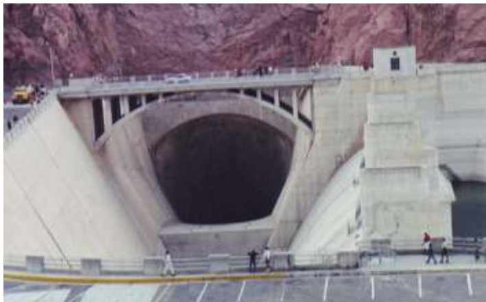
Hoover Dam spillway tunnel repair 1942
