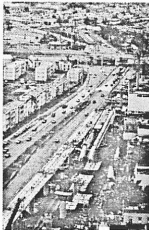
Single Track along PR-5
