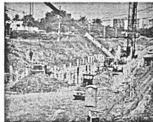
Retained Cut Section Concrete Piling
