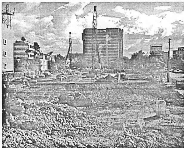
Pile driving at Centro Judicial
