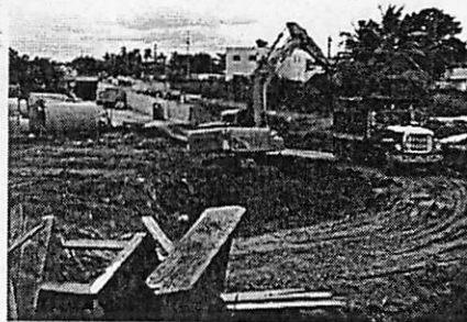
Demolition of Colectora Central Detour
