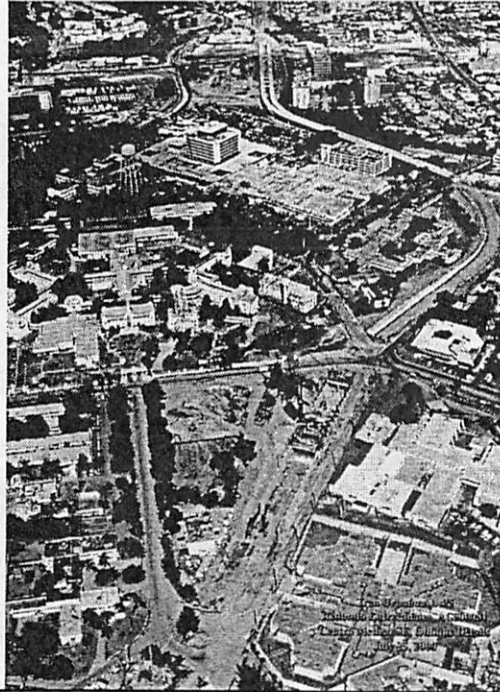
"Five Legs" intersection
