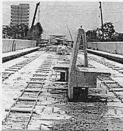
Las Lomas Bridge looking towards STTT
