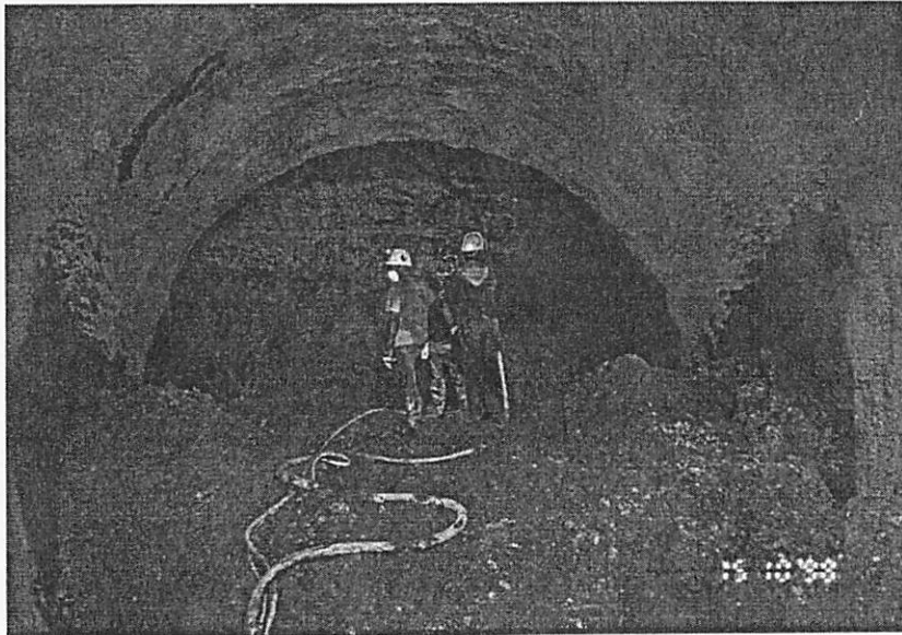
Figure 14. Heading of Carolina Left NATM Tunnel
