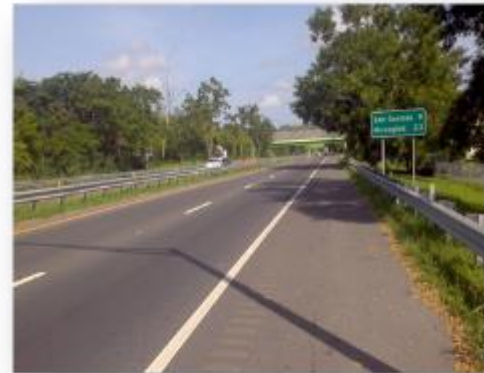
Pavement Rehabilitation and Safety Improvements (AC-200247, Sabana Grande)
