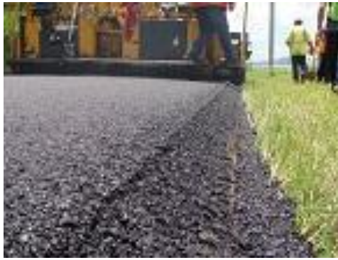
Figure 1. Safety Edge angle at PR-184 Yabucoa, PR
