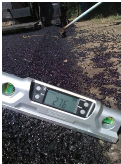
Figure 9. Angle of 27.6 achieved at the edge of the road
